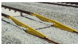
Longitudinal laying with temporary track (VPR)
