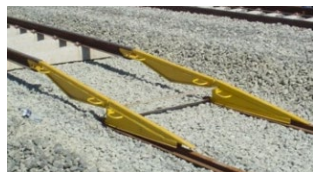
Longitudinal laying with temporary track (VPR)
