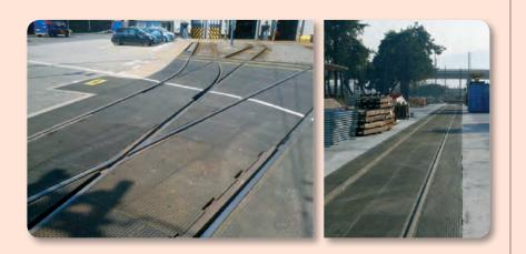
» These crossing panels are designed for emergency access and maintenance access onto, or across the tracks, and for use in depots, sheds and relief roadways - see the Stromferry images on the back of this leaflet.
