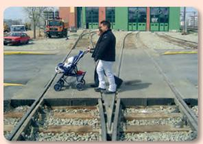
» Pedestrian panels are designed to provide safe transit for foot traffic across the tracks and have been supplied to rail networks throughout Europe, Australia and New Zealand.
